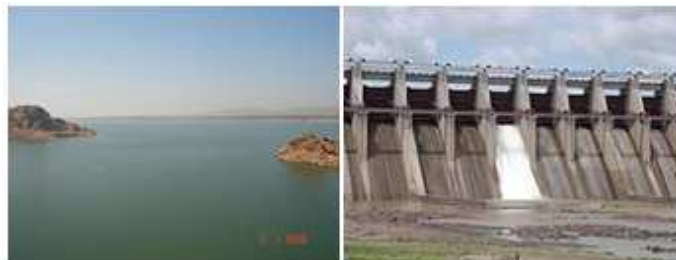
Fig. (a) Bansagar Dam Upstream (b) Bansagar Dam Downstream
