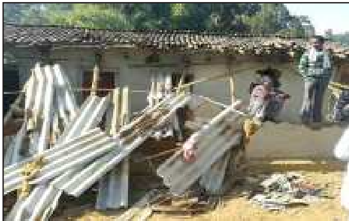
Fig. 1 - Devastation caused by 32 elephants entered the village & broken houses. (Dated – 11.03.2016 e-paper Patrika)
